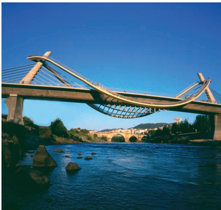
The Millennium Bridge
